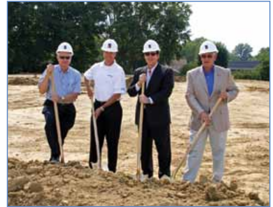
Groundbreaking for Galbraith Professional Building on Aug 30th. From left to right, Dick Kent (Trustee), Greg Hopkins (PPS owner), Dutch Cambruzzi (Camden Homes) and Cliff Bishop (Trustee).
