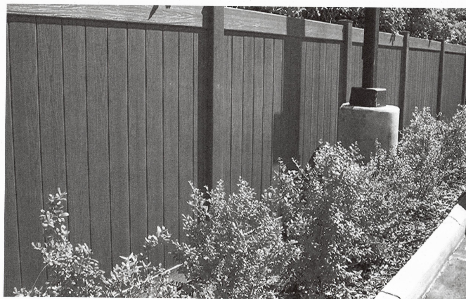
SCREEN FENCE TO BE STANDARD BROWN AS SHOWN IN ABOVE PHOTO. 6' HEIGHT PVC (VINYL) FENCE (SOLID FENCE 6' HEIGHT WITH 2' LATTICE ABOVE AS SHOWN IN PHOTO BELOW), BASIS OF DESIGN: MILLS FENCE CINCINNATI
