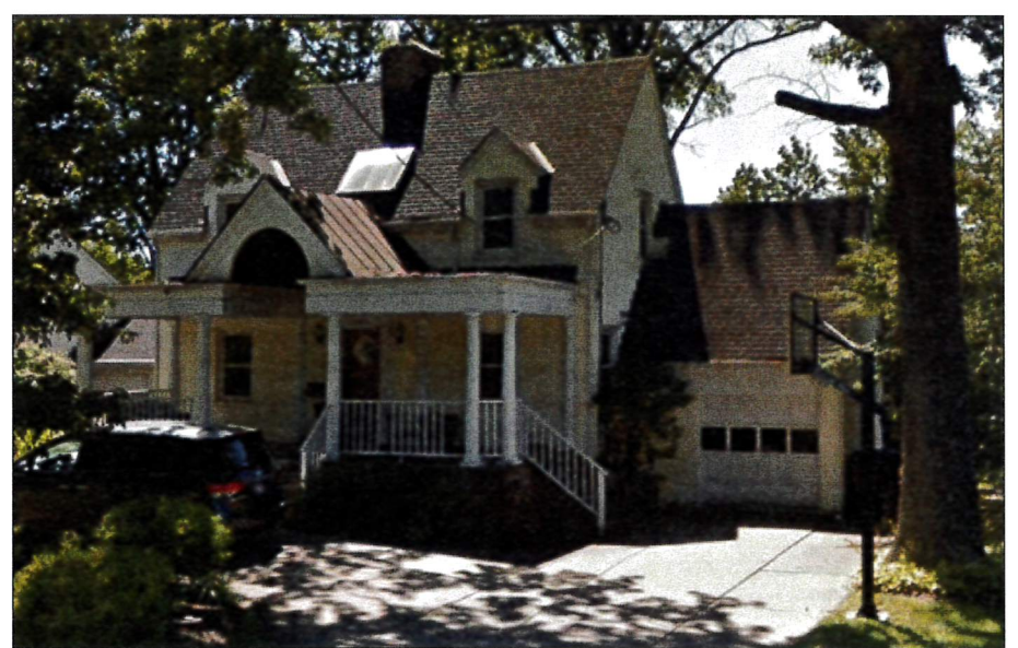
2 3 EXISTING FRONT PHOTO
