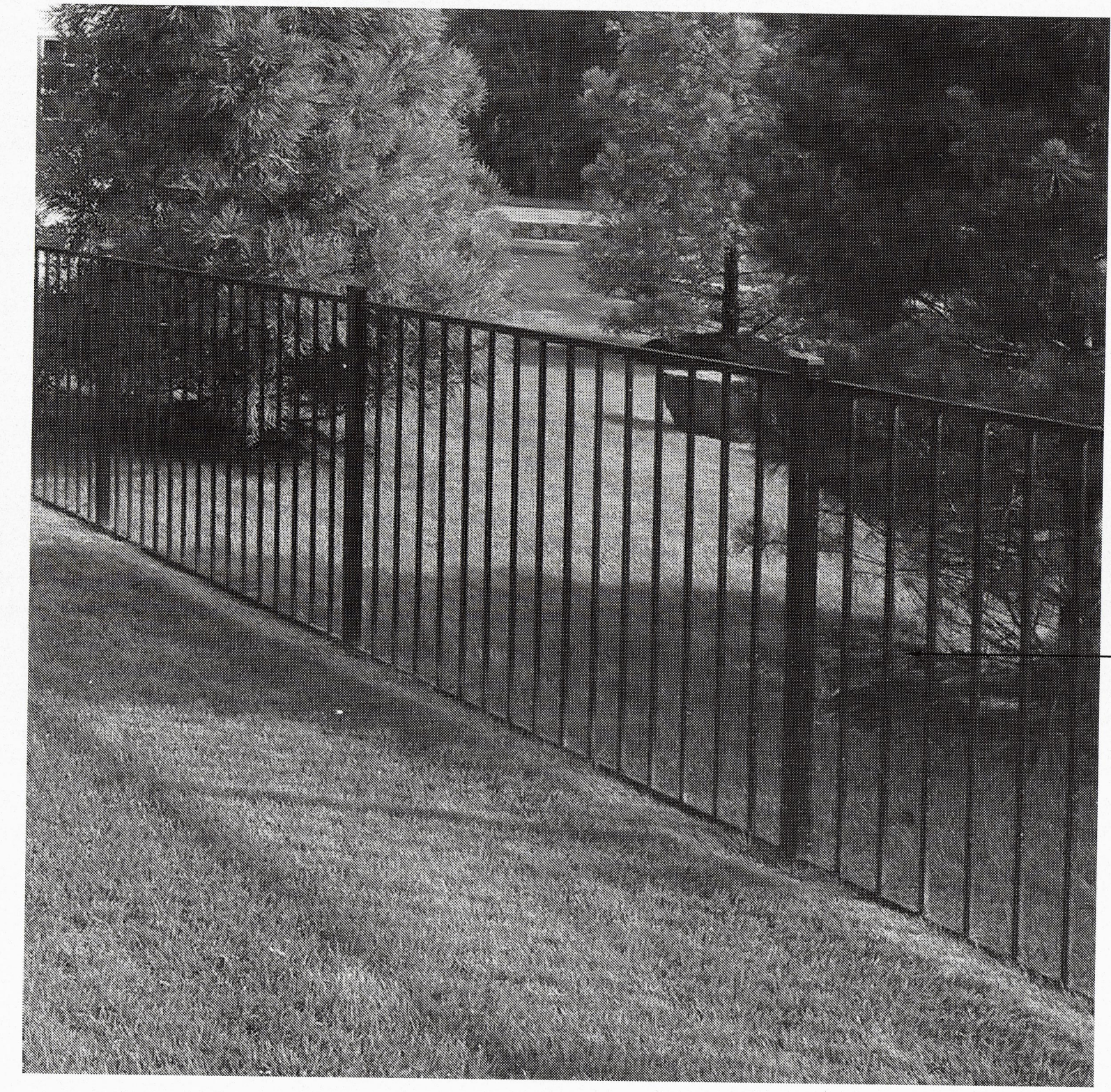
PROPOSED FENCING, BASIS OF DESIGN: FREEDOM (ACTUAL: 4-FT X 6.02-FT) STANDARD EASTON BLACK ALUMINUM DECORATIVE METAL FENCE PANEL
