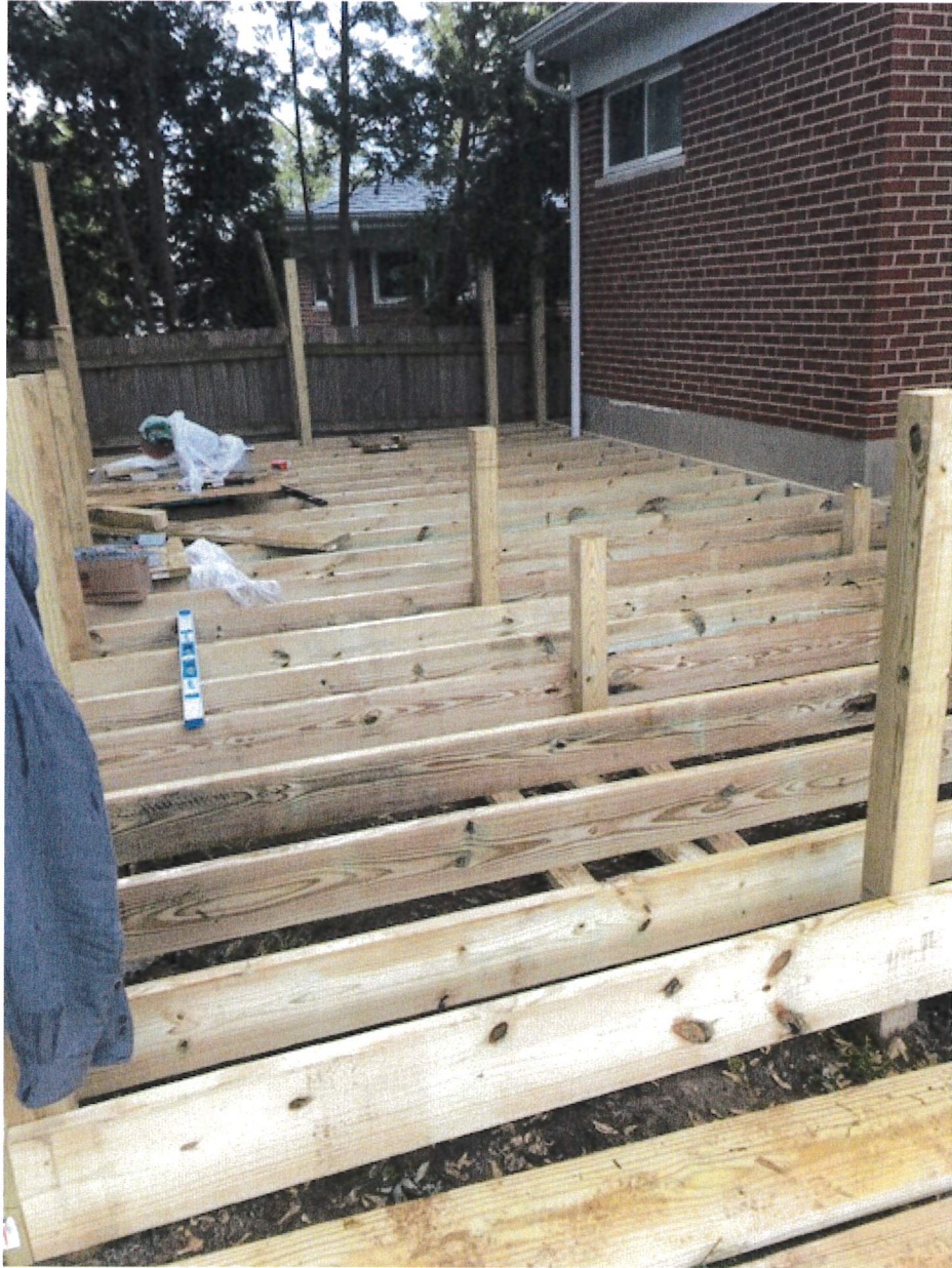
New deck joists while building
