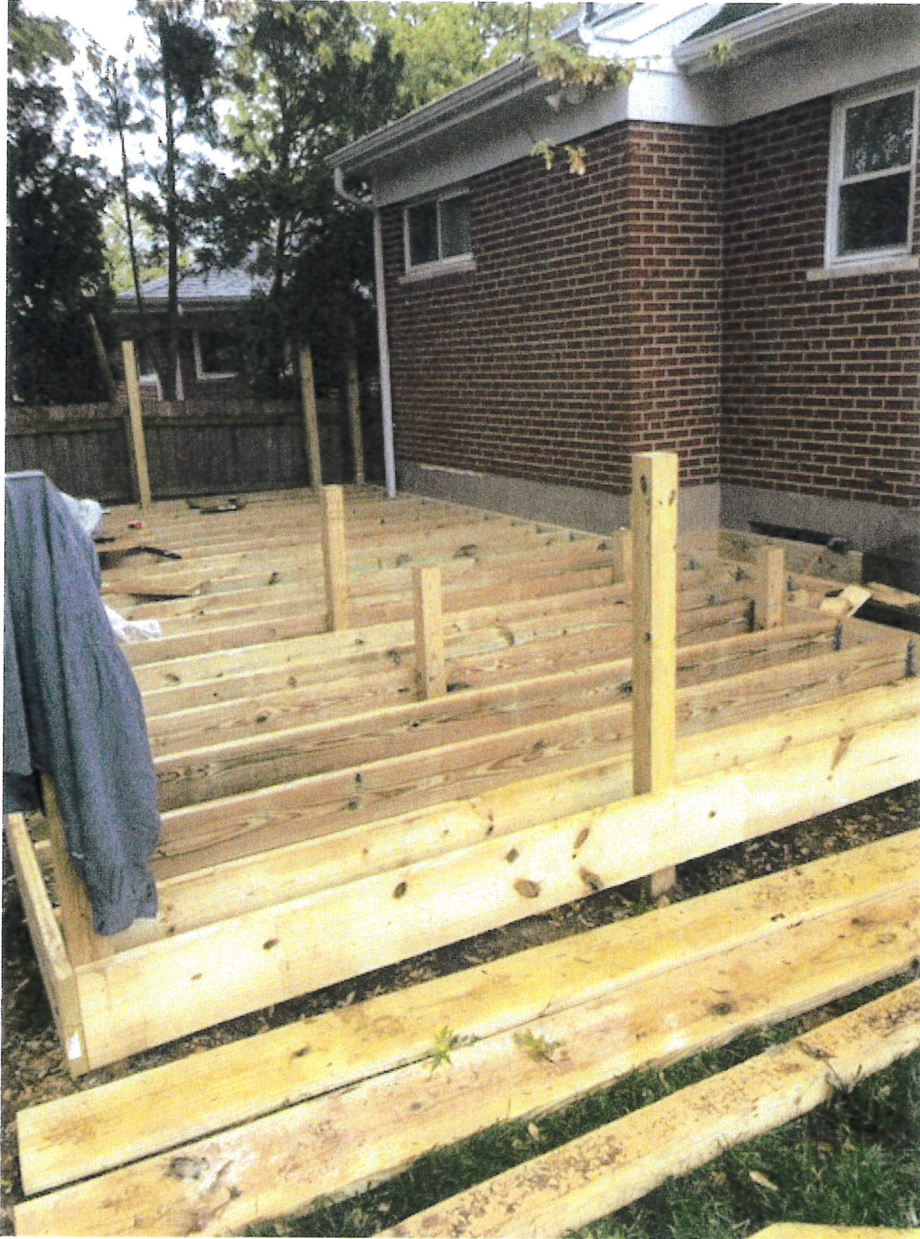
New Deck supports.
