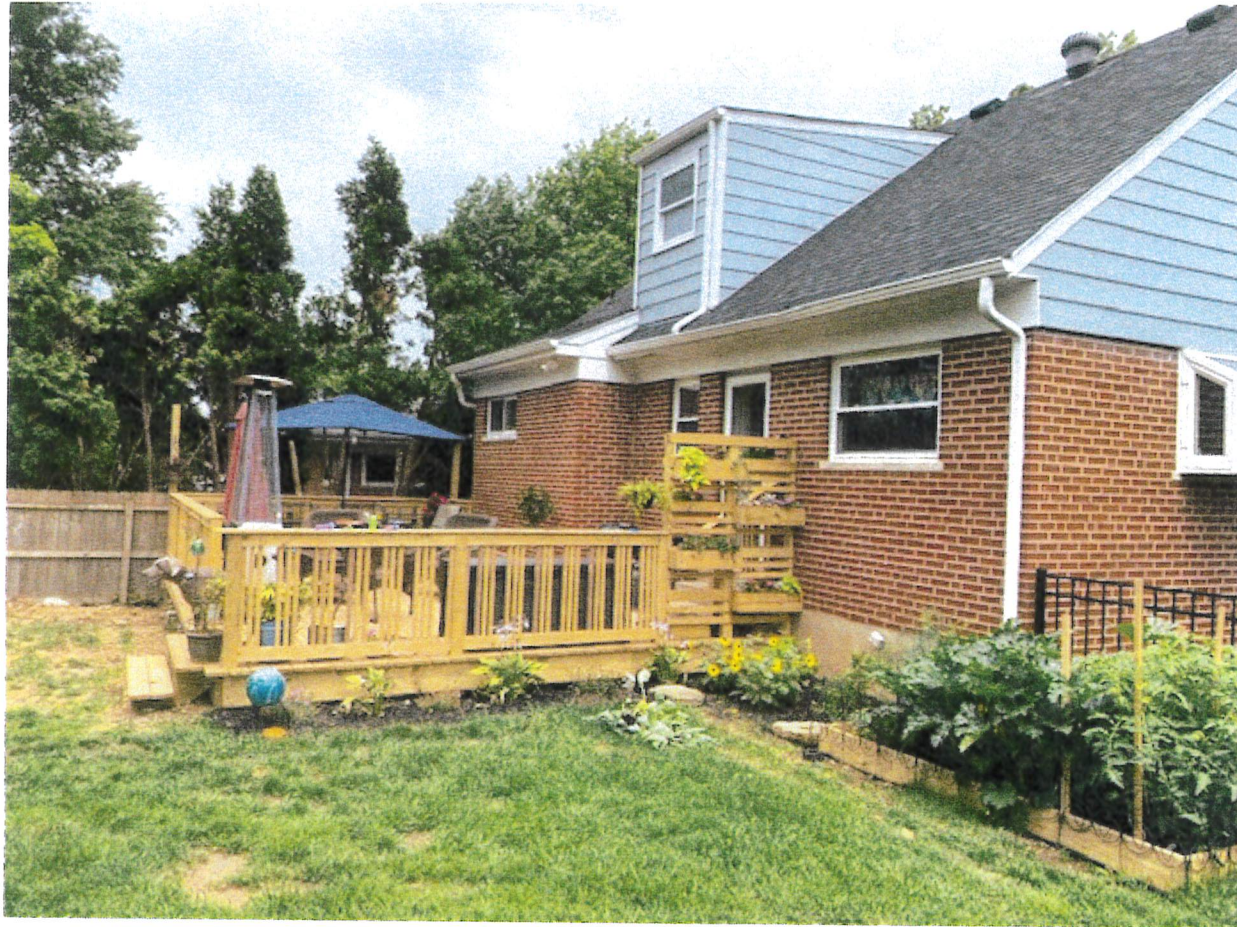
Completed deck Taken from inside fence on Styrax side of yard.
