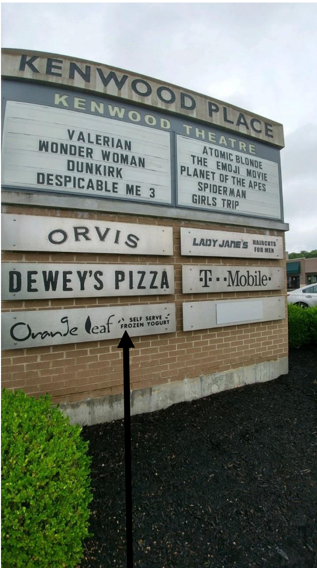
South Sign - North Elevation Panel location
