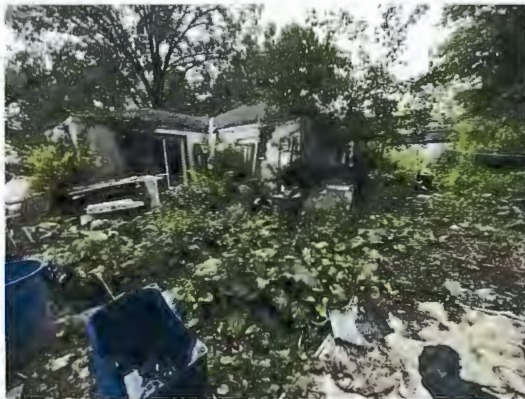
Rear of house 7/10/24
